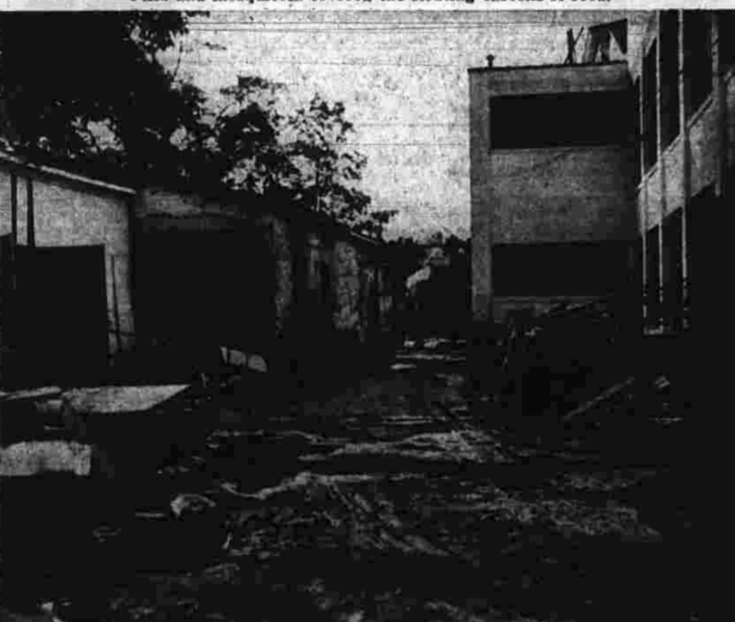
The flood waters wrecked havoc to this part of the storage area.
